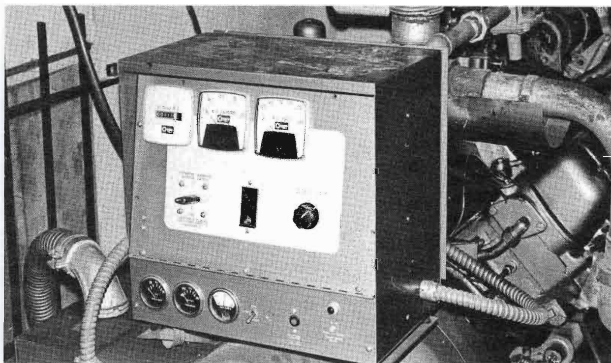
Fig. 3 Operation of the 50,000 Watt generator is completely automatic. Failure of any one of three phases of the commercial power will start the unit. When the power returns to normal, the generator will continue to run for about five minutes and then shut down. (Note the security bars over the air intake at left.)
